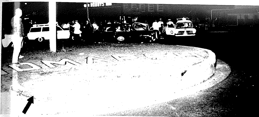
Fig. 8.14 Roundabout struck by the car shown in Figure 8.15. Arrow shows point and direction of impact.
