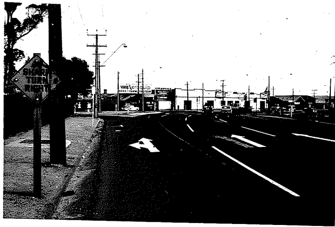
Fig. 14.3 Warning sign left in position after changes to the road layout.
