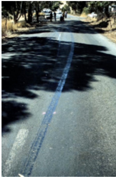
Figure 6.7.1 Tyre yaw marks in bleeding bitumen
