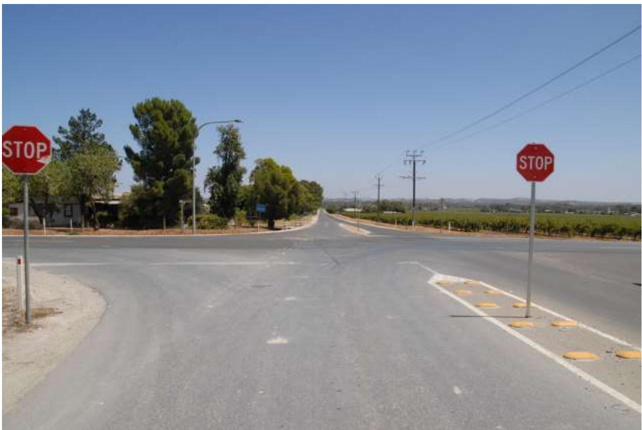
Figure 3.7 Penrice Road through the intersection with Stockwell Road in Light Pass in 2018, facing west from the eastern side of the intersection
