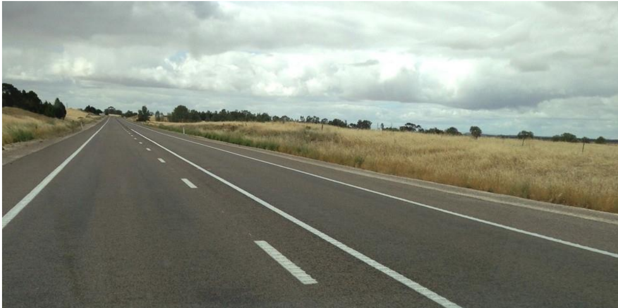
Figure 2.2 Wide centrelines on the Duke's Highway
