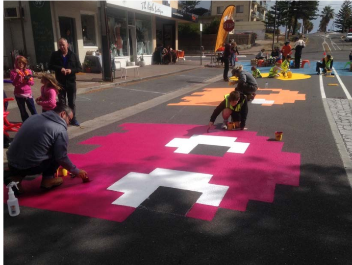
Figure 3.1 Road Mural being painted by the community in Jetty Street, Grange (April 2017).
