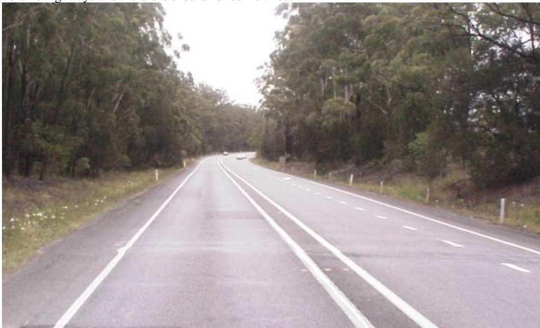
Image 2 - 0.5m wide painted median – Pacific Hwy – north of Port Macquarie
