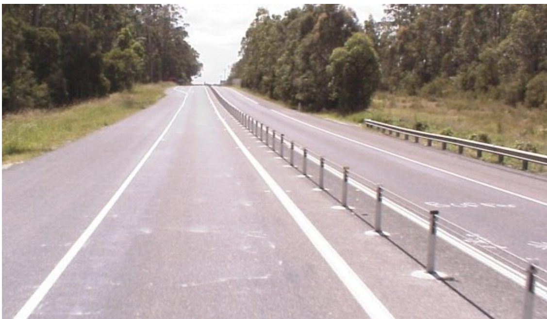
Image 5 - 2.0 metre wide Wire Rope Safety Barrier median – Pacific Hwy, at New Italy
