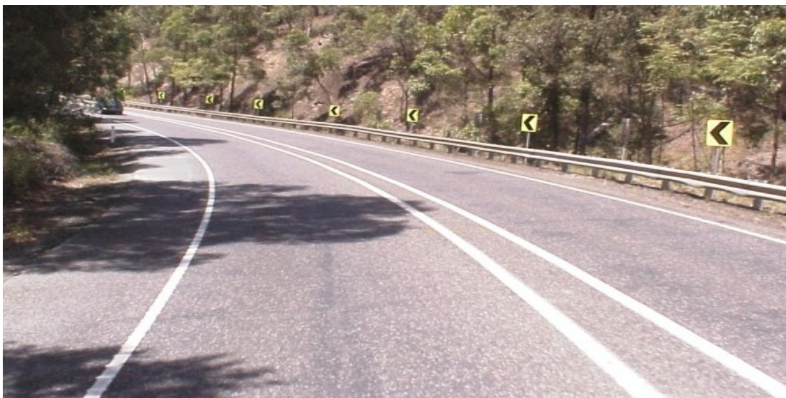
Image 4 - Variable width audio-tactile profile median - Pacific Hwy south of Urunga
