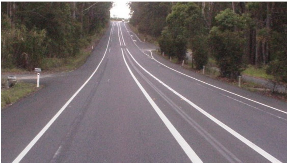
Image 3 - 1.0m wide painted median, Pacific Hwy south of Urunga (note old line marking)
