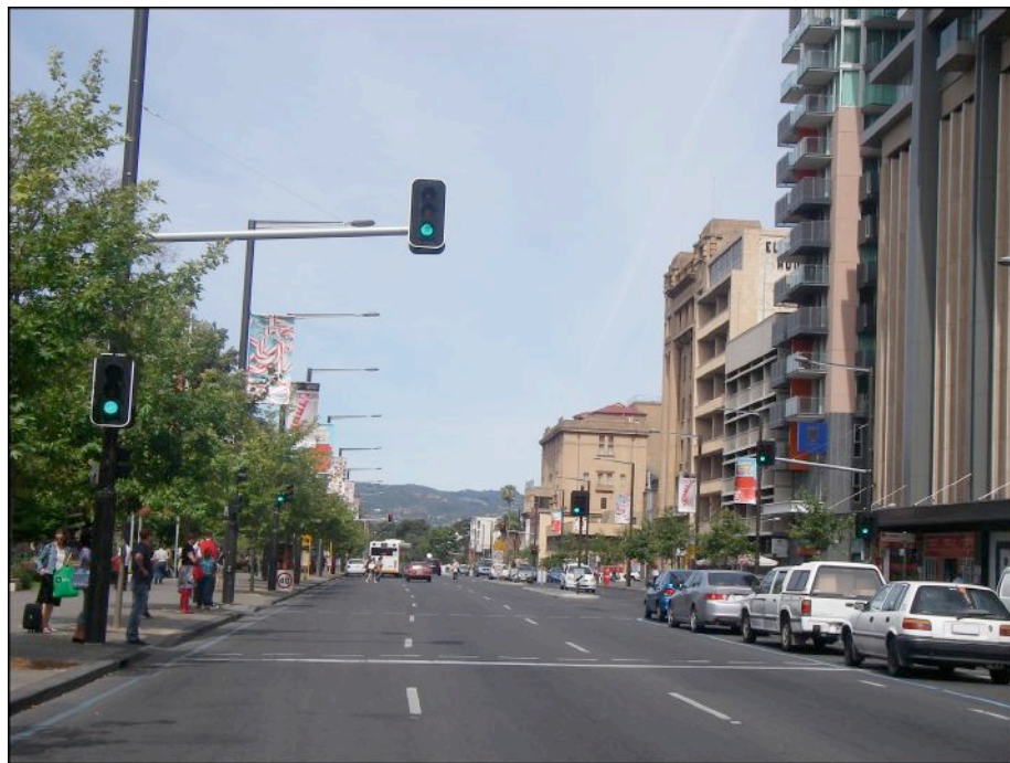
Figure 3.3 Mast arms on approach and departure of a signalised intersection, Adelaide
