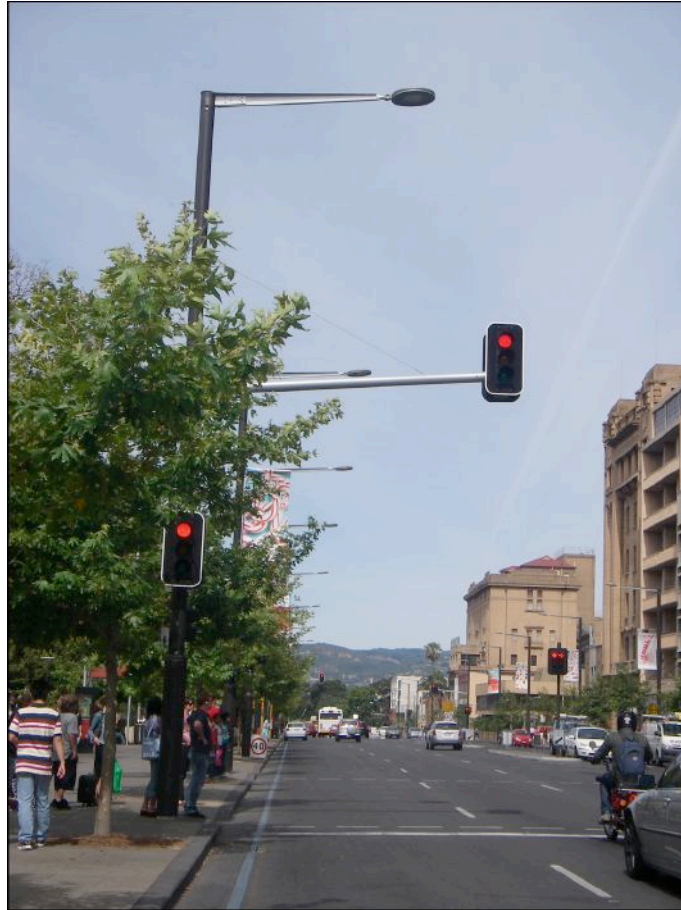
Figure 3.1 Combination mast arm at a signalised intersection, Adelaide CBD
