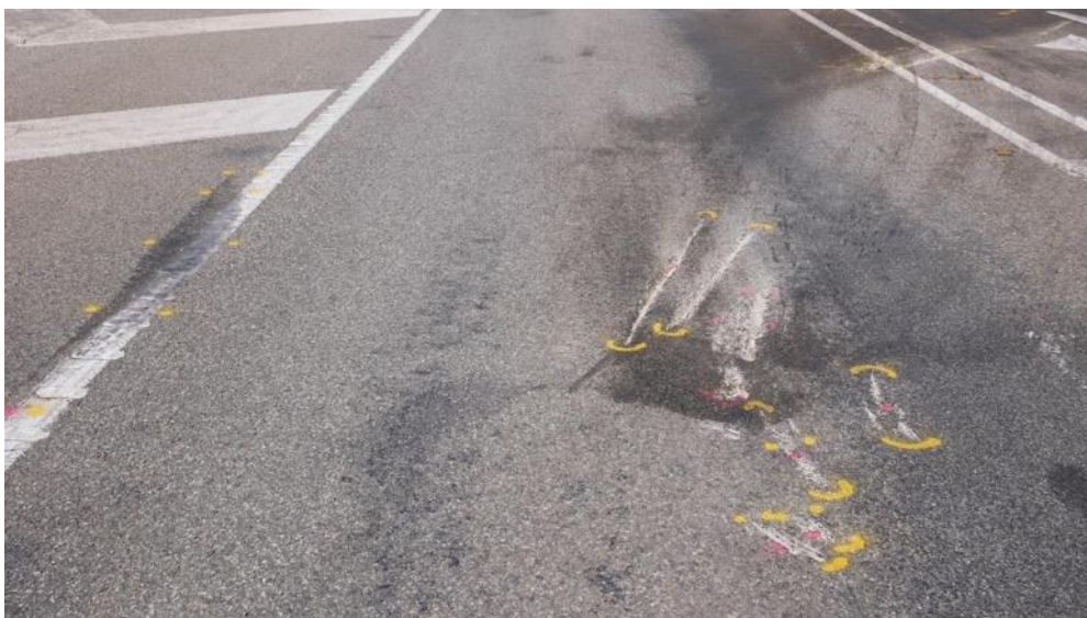
Figure 2.3 Example of scrape marks on a road close to the point of impact from collision forces causing parts of the vehicle to come into contact with the road
