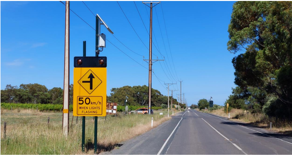
Figure 3.17 Westbound major road speed advisory sign, which was installed under overhead powerlines
