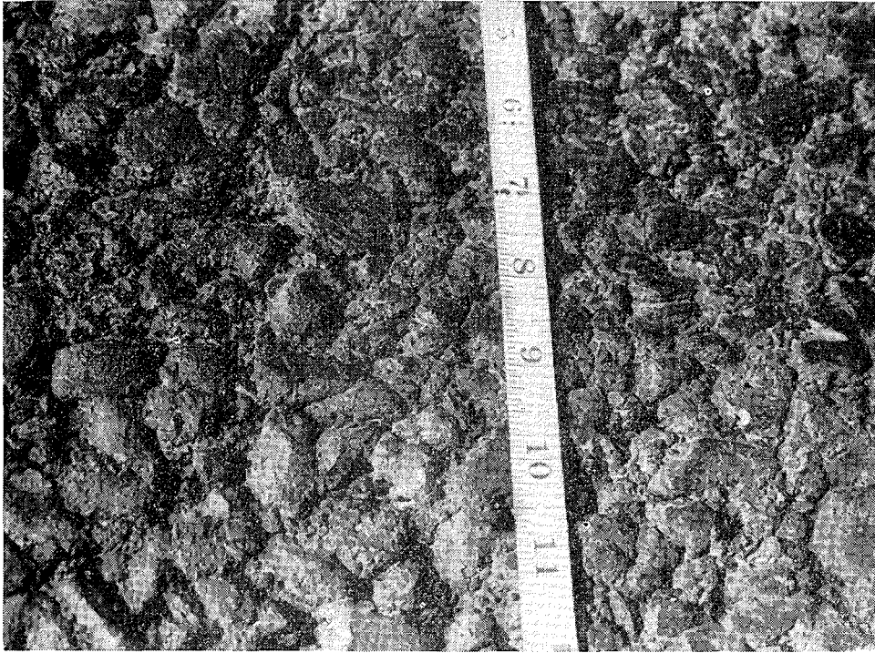
Fig. 10.13—Detailed view of the skid mark and road surface shown in Fig. 10.12. The tape measure shows inches
