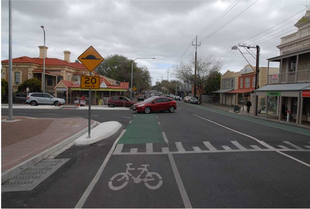
Figure 3.2 Plateau treatment implemented at a high crash risk intersection in Kent Town, Adelaide.
